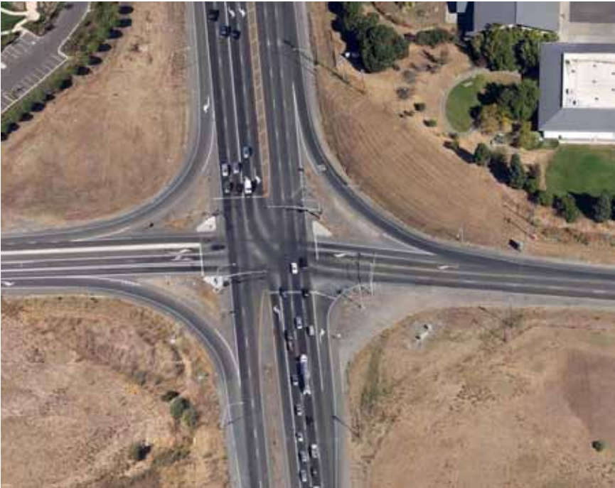
Existing Condition: SR 29/Airport Boulevard/Jameson Canyon Road
